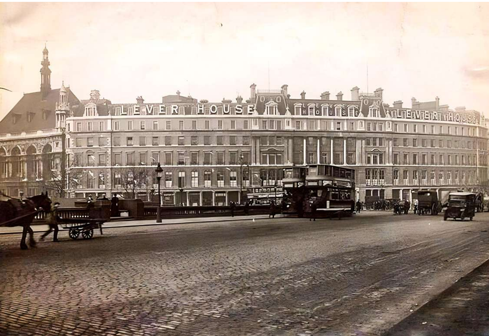
| Lever House, London, UK (1922, Pre Unilever House Construction) |
